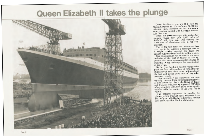
This is an extract from a Siftips magazine circa 1967 where the QEII super structure was welded with SIFMIG 5356
